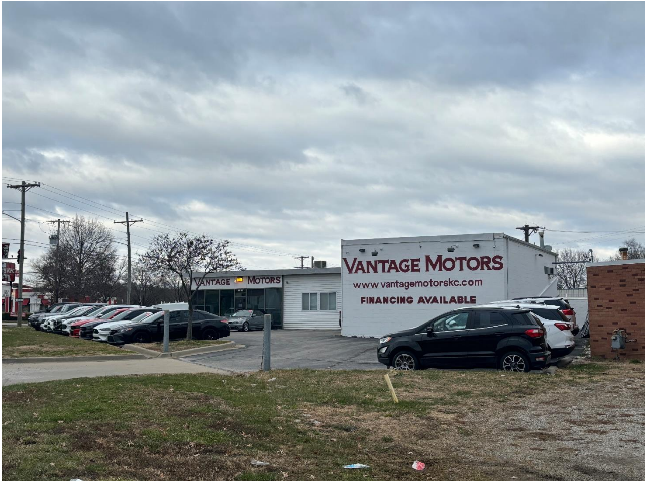
Facing north from the south edge of the lot
